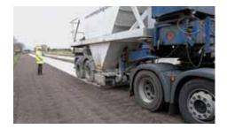
into the mix from nozzles in the crown of the Wortgen's rotovating drum chamber. All the ingredients were thoroughly mixed to reconstitute and strengthen the old base course.
